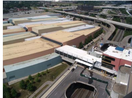
Designers replicate convention center roof lines for lighting design in the new Battelle Grand ballroom.
