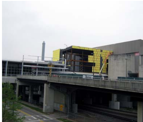
Construction of the new north hall pre-function structure over the existing bridge deck and railroad track.
