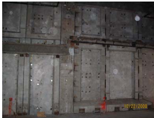
Discovery of welded steel embeds in the existing exterior precast wall.
