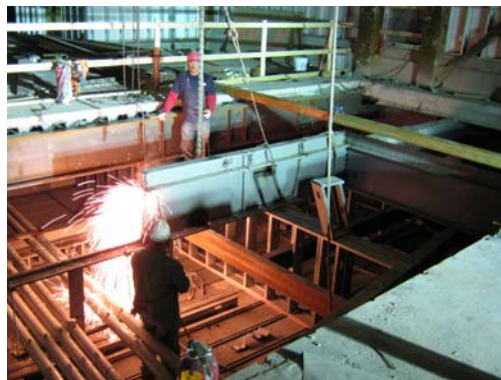
Construction of the new north hall pre-function structure over the existing bridge deck and railroad track.
